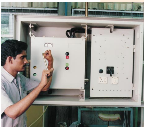
Emergency manual spring charging in the event of loss of control supply
