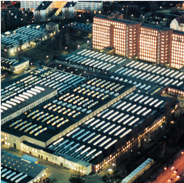
Switchgear Factory in Berlin, Germany
