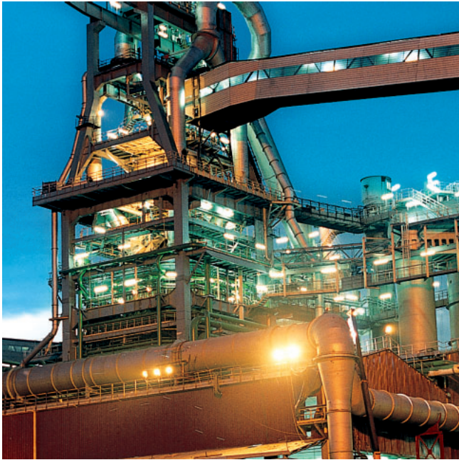
Industrial application: Refinery
